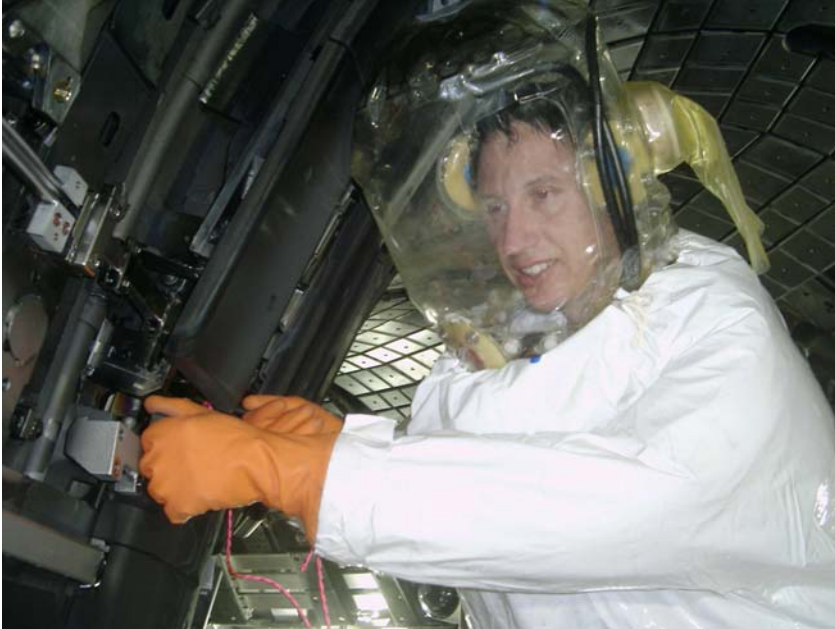
Figure 3.4: Manual work inside the JET Torus.
