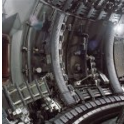
Figure 2.7: Interior view of the JET vacuum vessel The inside of the vessel is about three metres high
