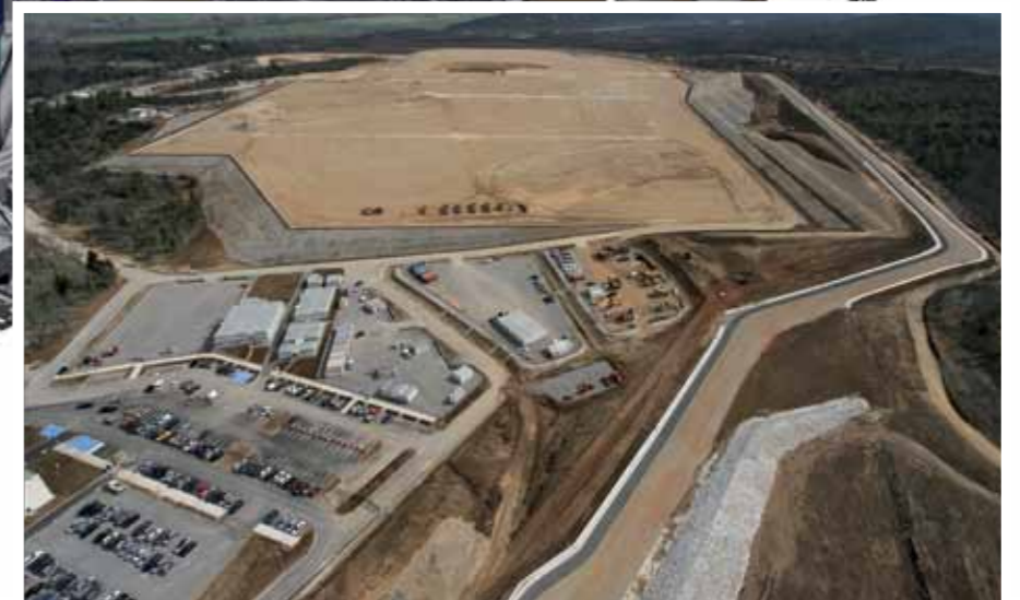
The ITER construction site at Cadarache, France
